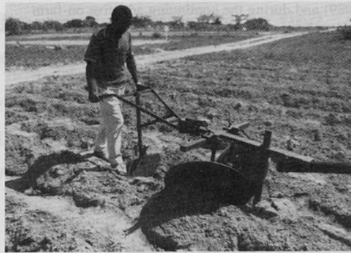
Photo 2: Disc ridger in re-ridging and ridge-tying mode
